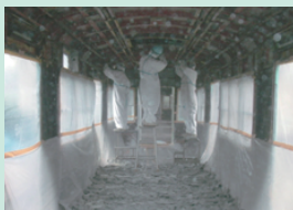
Removal of asbestos
