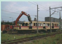
Disassembly of car body
